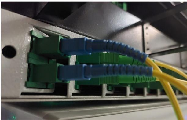
No conectes fibra SC/UPC con patch SC/APC
